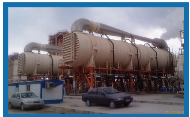
Complete Design three 4000 m 3 /day MED- TVC Units - Kavian Petrochemical Co,
