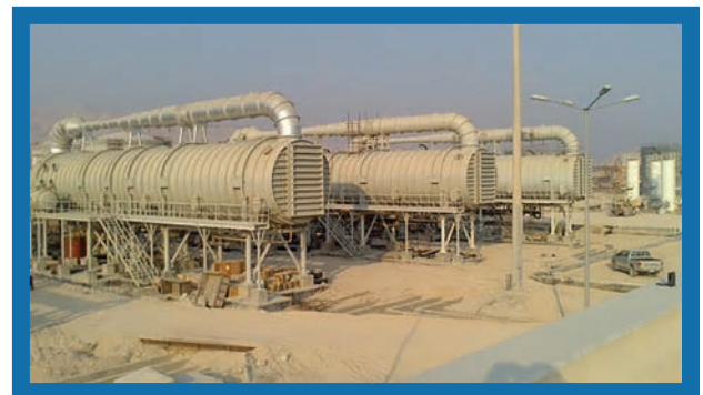
Engineering supervision MED- TVC Units - phase 22,23 and 24 of South Pars gas field, Petrosina Aria
