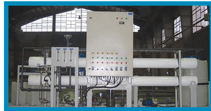
EPC of 160 m 3 /day RO Units - FZACO
